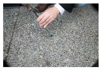
6. Drill the holes to a depth of 1-5/8" (as suggested by the anchor manufacturer) – ensure drill is level, straight up and down so that the anchor inserts correctly.
