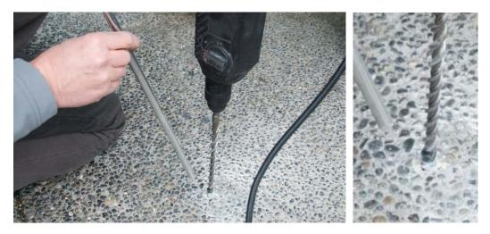
8. Insert concrete anchor. Hammer the anchor with the supplied post tool to expand the anchor's base, securing it to the concrete.
