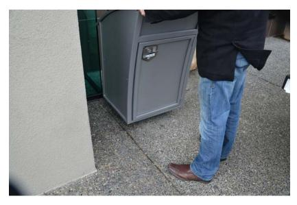
2. Mark with a felt pen where the fasteners need to me positioned, through the bolt hole locations in the base of the receptacle.
